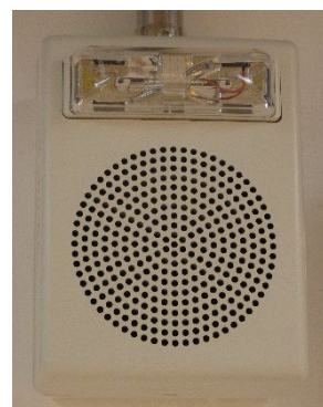
Figure 1 ESB Fire Alarm Light & Horn Combination
