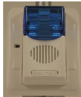
Figure 3 TGMS Alarm Light & Horn Combination
