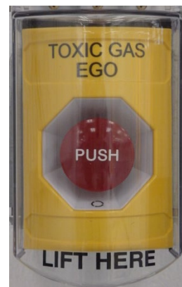
Figure 6 Emergency Gas Off (EGO) Push-Button
