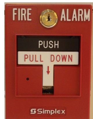
Figure 5 Typical Fire Alarm Pull-Station
