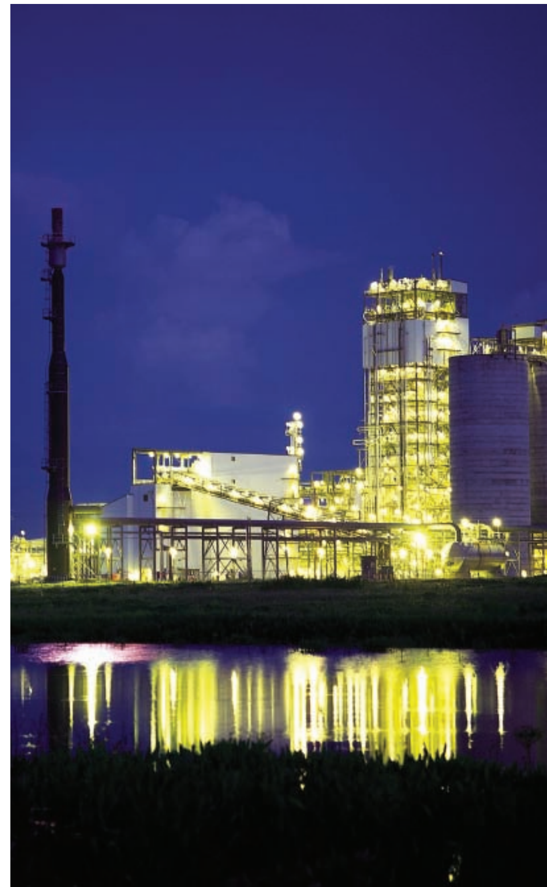
A nighttime view of a large coal-gasification plant. Vanderbilt researchers are studying coal-combustion residues to help the Environmental Protection Agency regulate power-plant emissions in ways that will protect human health.
