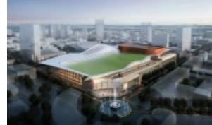
Downtown Nashville's new convention center will feature a four-acre green roof, which is scheduled to be completed by the end of March. The green roof, which is being installed by Landscape Support Services of Murfreesboro, is being put in place to avoid urban storm-water runoff and as an added benefit may provide some insulation to the convention center.
