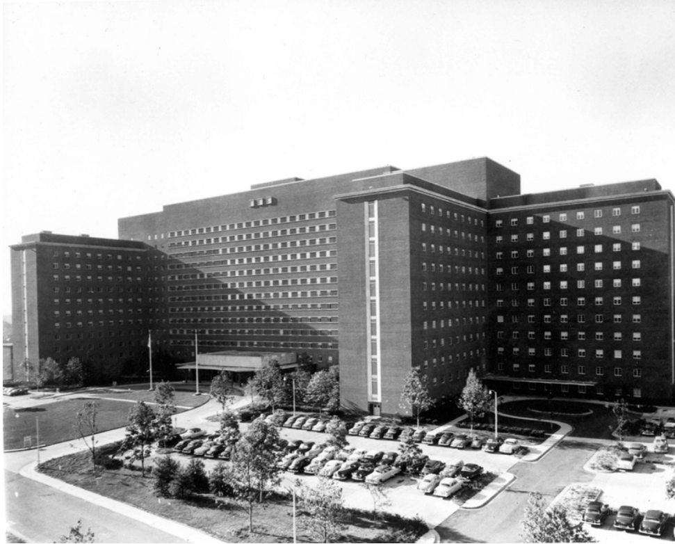
Fig. 1. Exterior view of the Clinical Center NIH circa 1953. Source: Collection: Images from the History of Medicine; Record UI 101441174.
