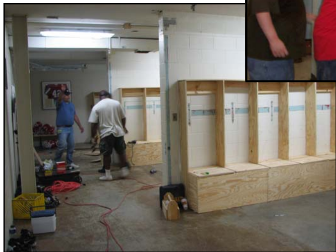
Lockers being installed at Glenclyff High School
